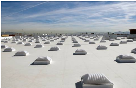
Skylights provide natural daylight
